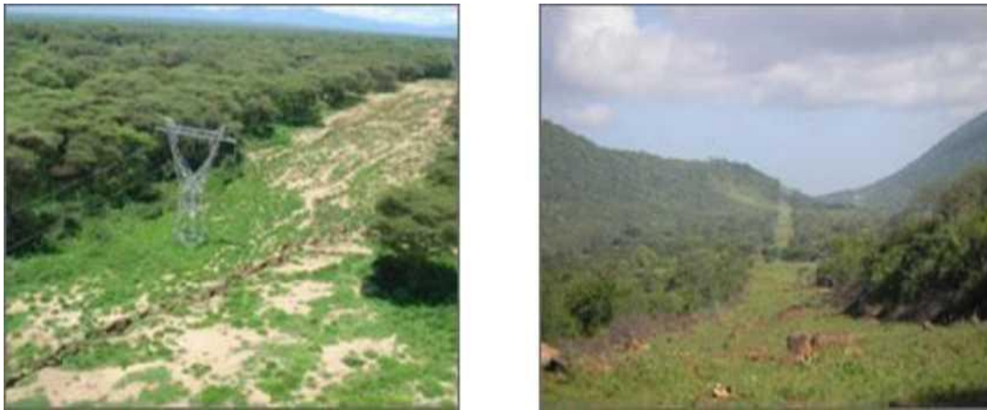
Figure 3. Existing power line trace (L) and a newly cleared route corridor(R). Source: KETRACO (2007).
