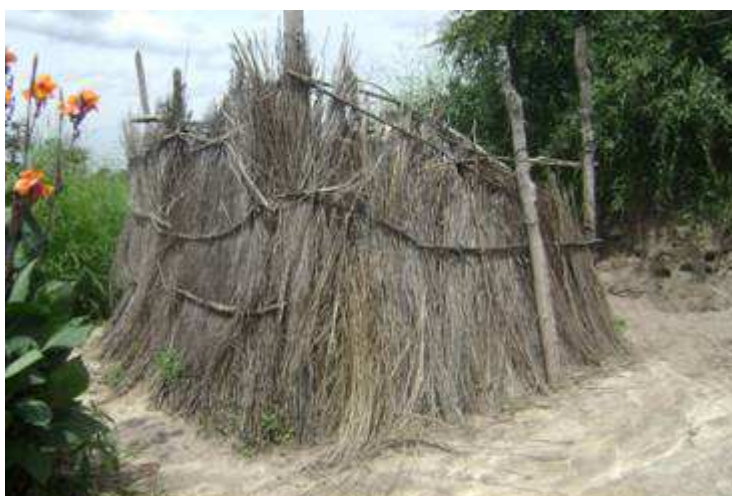
Figure 5: Existing situation to some of schools in Kahama district. Photographs are taken to each action as supporting evidence to decision makers.
