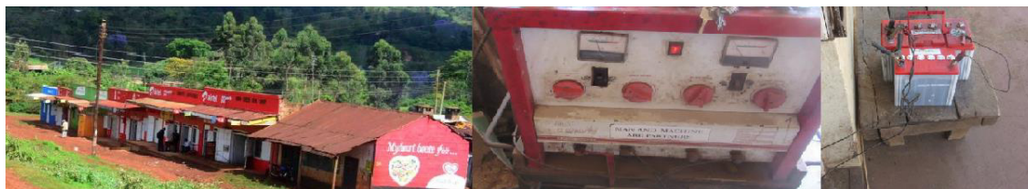
Fig. 7. (a) A typical rural shopping centre; (b) A battery charging system
